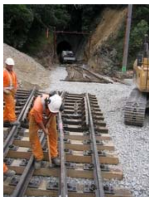
Figure 5: Johnsonville Tunnels infrastructure modifications
